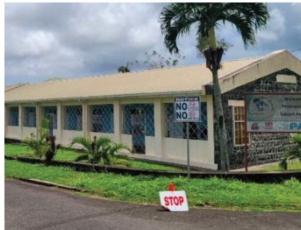
Princess Alice Hospital in mainland Grenada suffered minor damage. Photo PAHO 2024
