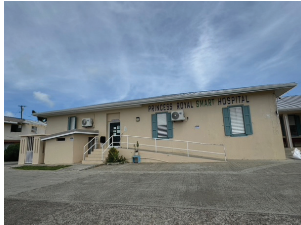
Princess Royal Hospital the only one serving Carriacou and Petite Martinique (8,000 people) lost 70% of its roof sheeting, the incoming rains left the facility non-functional. Severe damage to the nurses' and doctors' housing impacted operations. Photo PDNA team
